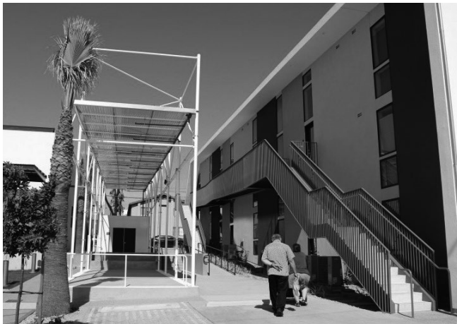
Figure 5. "Living Rooms at the Border" Casa Familiar Development, Estudio Cruz, San Ysidro, Ca. Image credit www.casafamiliar.org/livingroomsattheborder/
